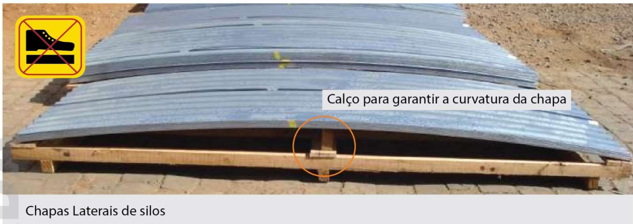
Figure 13 - Correct way to store side panels on site.
